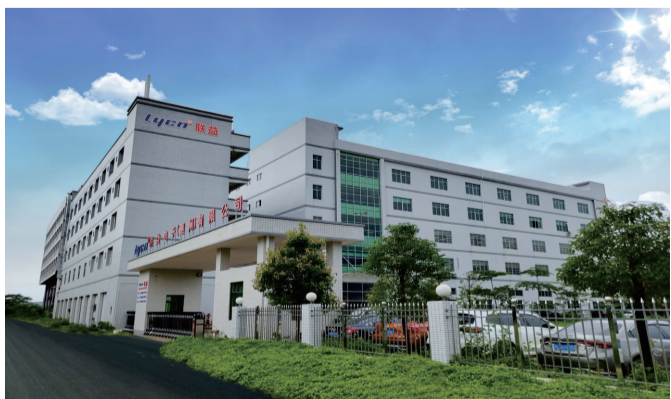
总部基地(惠州) Headquarters Base(HUIZHOU)
